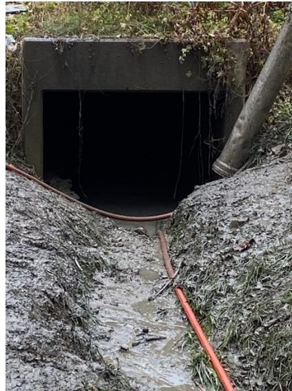
The pictures show an example of why developing an ordinance and educating the public about stormwater drains is important. This is a stormwater culvert that Ace recently cleaned out and it was filled with debris. When storm drains become blocked like this, it can lead to flooding and standing water. These kind of materials should not be in a storm drain.
